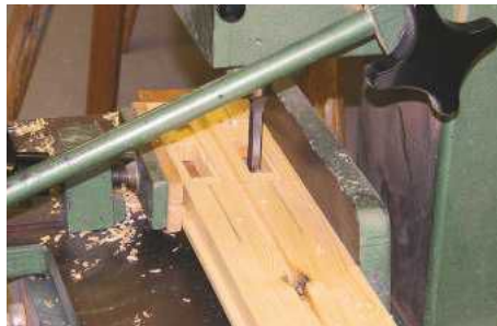
▲ Pic.5 A combination of router and mortising machine forms the recesses for the pulley wheels
